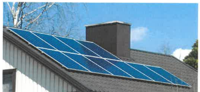
Solar panels are creating energy for this house.
