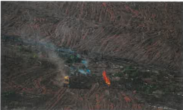
This bulldozer is clearing the trees out of the way.
